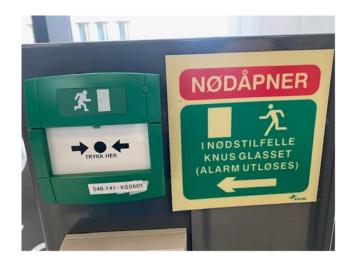
**Emergency** opener to be used for evacuation if the door is locked
